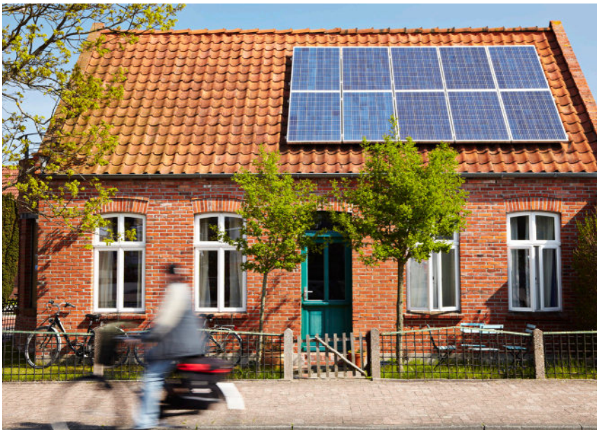
Social influence can be a powerful tool. Research shows that installing solar panels on your home increases the odds that neighbors will do the same.
